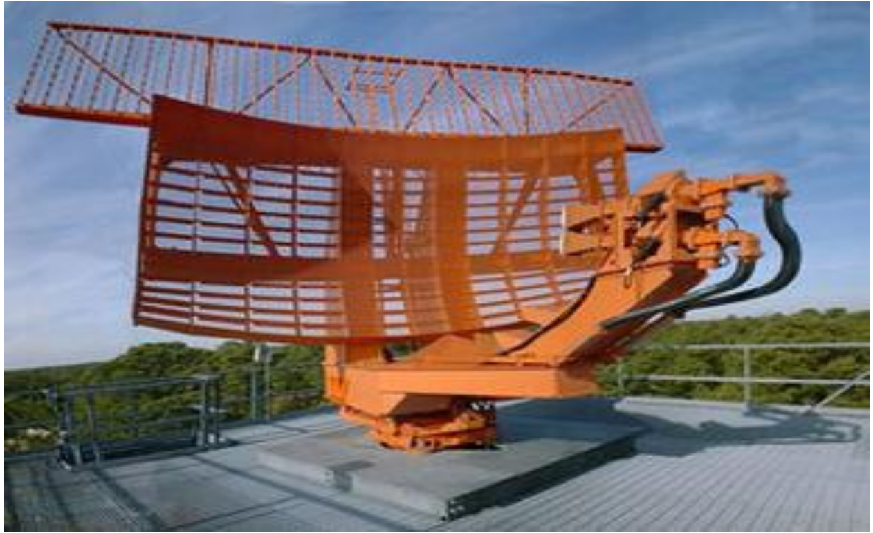
Airport Surveillance Radar
